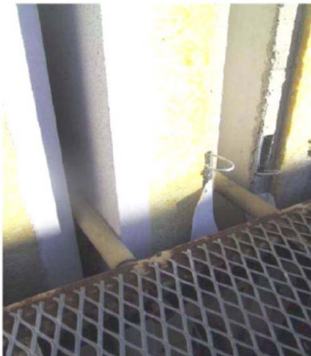
Figure No.3 Wall securing during storage. Attention should be paid that the wedges are coated with non-soiling, water non-absorbent material
