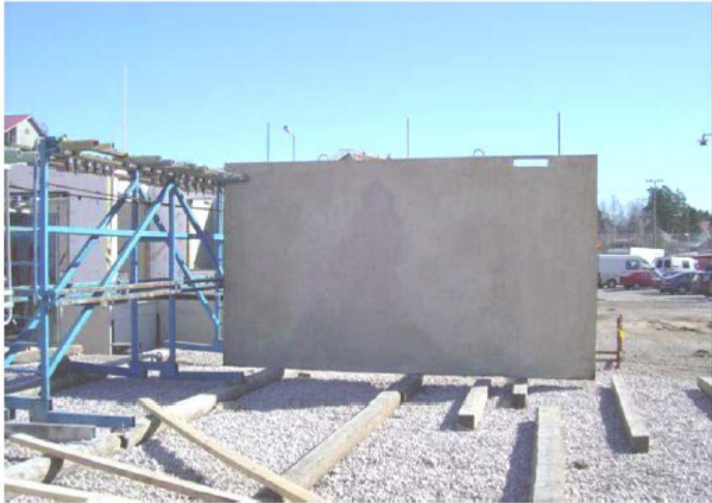
Figure No.2. Storage of walls. Attention should be paid to the size of the wooden rest bars!
