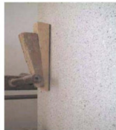
Figure No.2. Storage of walls. Attention should be paid to the size of the wooden rest bars!
