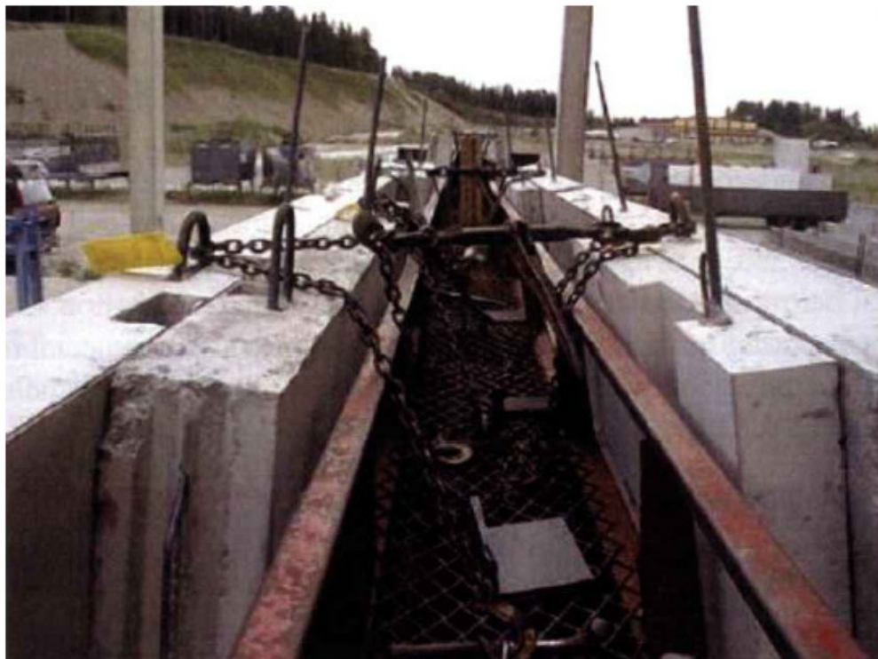
Figure No.4 One-layer wall slabs stored in pyramid and secured.
