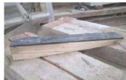
Figure No.3 Wall securing during storage. Attention should be paid that the wedges are coated with non-soiling, water non-absorbent material
